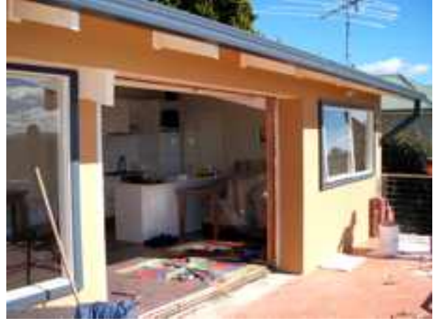
FIRST STEPS REMOVE DOORS AND FRAMES
