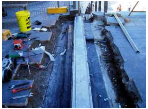
WE HAD TO CONTINUE DOWN THE STEPS TO FOLLOW THE CONSTRUCTION JOINT
