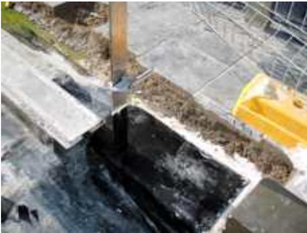
FLOOD TESTING WITH DYE WHEN PRACTICAL. "NO LEAKS"
