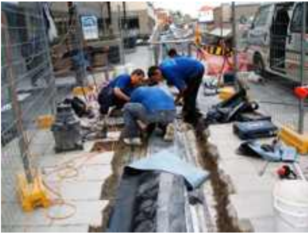
PROPER MEMBRANE TERMINATION REPLACES THE BLOB
