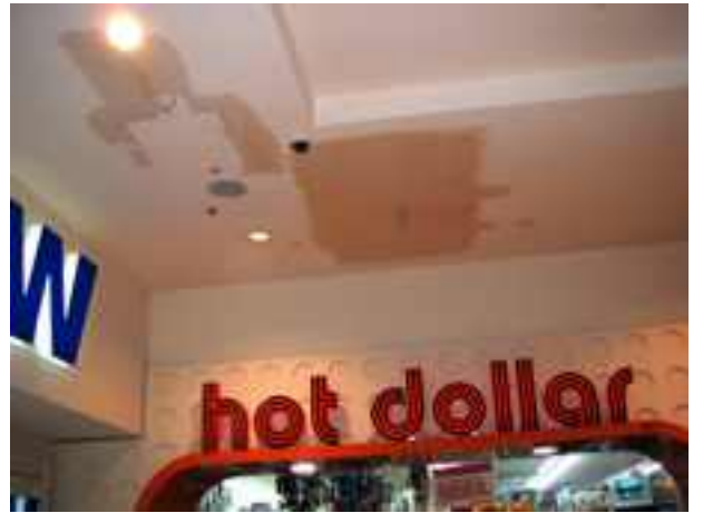
AND UNDER THE BLOB THE CONSTRUCTION JOINT
