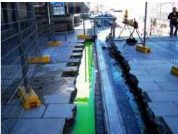
PVC MEMBRANE INSTALLED DETAIL WELDING NEXT
