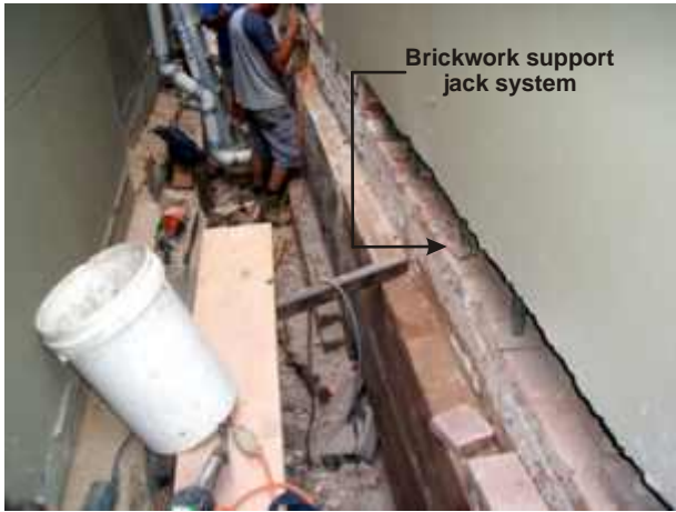
AIDING THE MEMBRANE TRANSITION
