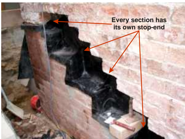
CAVITY STEP FLASHING AT THE OTHER END OF THE BUILDING
