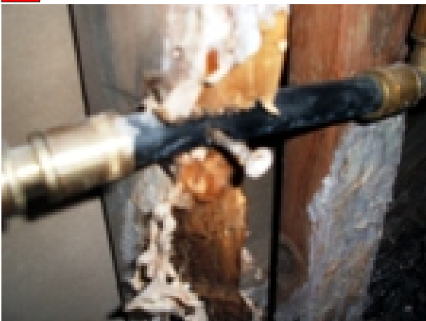
NAIL THROUGH WATER SERVICE
