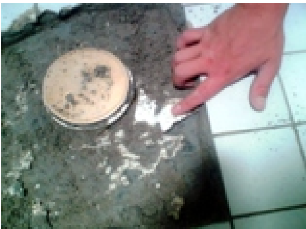
NAIL THROUGH WATER SERVICE
