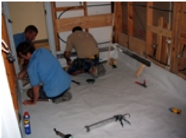
SLIP SHEET & REINFORCING MESH INSTALLED
