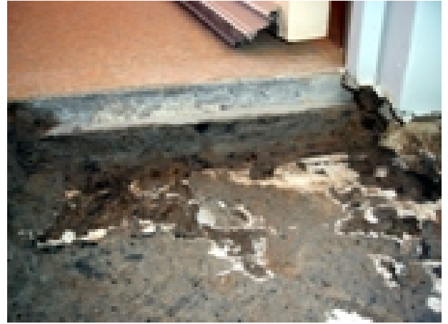
CORRODED STEEL DOOR JAMBS
