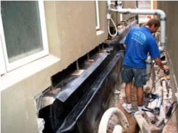
THE MAIN PVC MEMBRANE AREAS ARE INSTALLED
