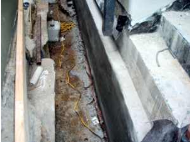
THE MAIN PVC MEMBRANE AREAS ARE INSTALLED
