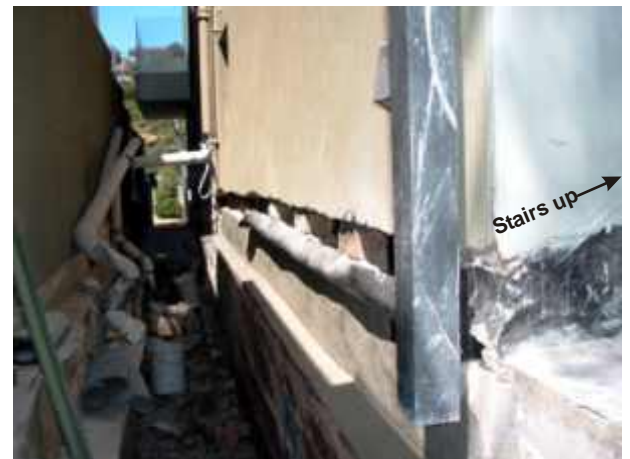
THE STAIRS ARE ENCAPSULATE & WELDED TO THE CAVITY FLASHING
