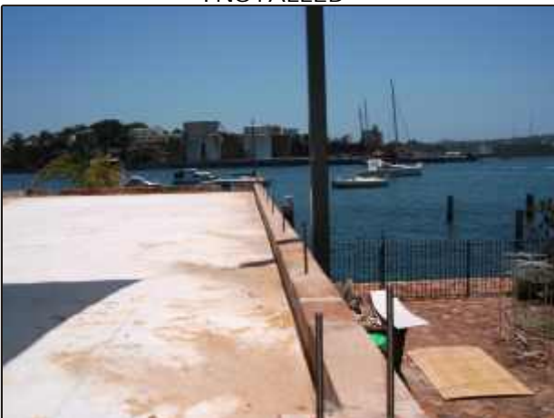
STAINLESS THREADED RODS INSTALLED
