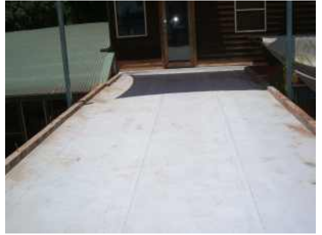
THE SLAB WAS GROUND SMOOTH & PVC MEMBRANE INSTALLED TO THE EDGES
