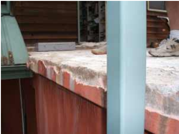
THE TIMBER CLADDING WAS STRIPPED TO INSTALL THE PVC MEMBRANE
