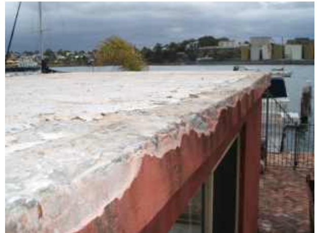
THE SLAB WAS GROUND SMOOTH & PVC MEMBRANE INSTALLED TO THE EDGES
