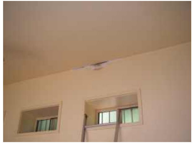
STRIPPING OFF TO START AGAIN
