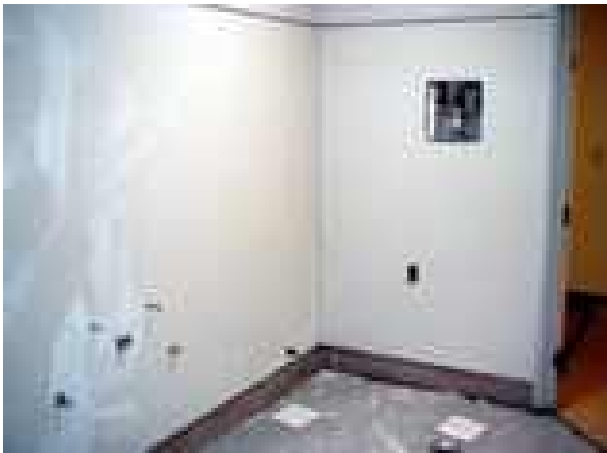
✓ VINYL FLOOR COVERING INSTALLED
