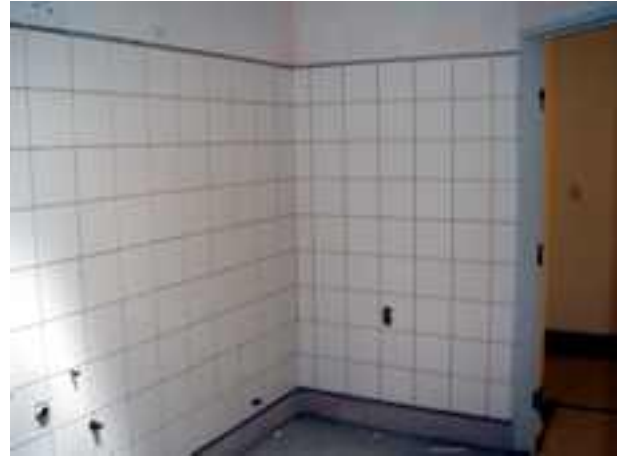
✓ LEVELLING TOPPING APPLIED FOR VINYL FLOOR COVER
