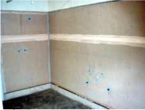
✓ GROUTING FINISHED WITH VERTICAL JUNCTIONS TO BE CAULKED
