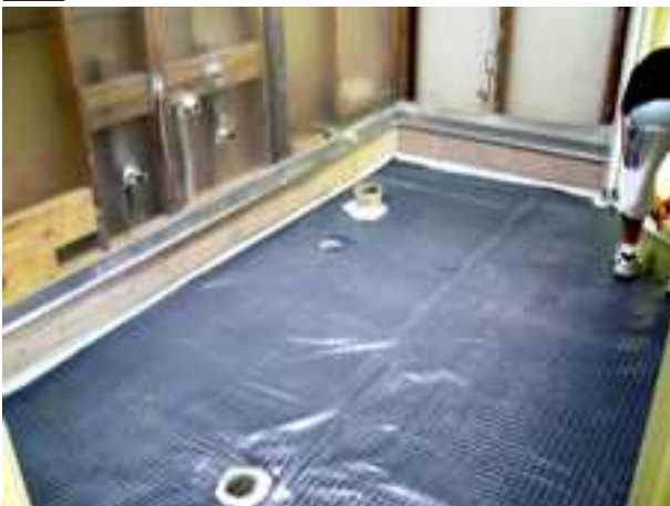
SLIP SHEET & REINFORCING MESH INSTALLED
