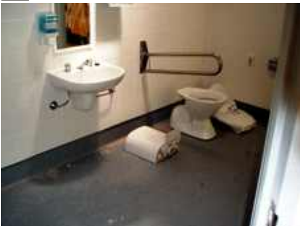
✓ NEW PAN IS INSTALLED
