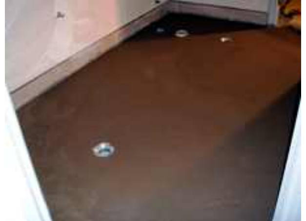
✓ PC ITEMS REINSTALLED IN THE ORIGINAL POSITIONS
