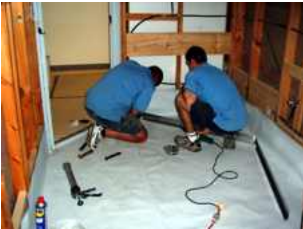
SLIP SHEET & REINFORCING MESH INSTALLED
