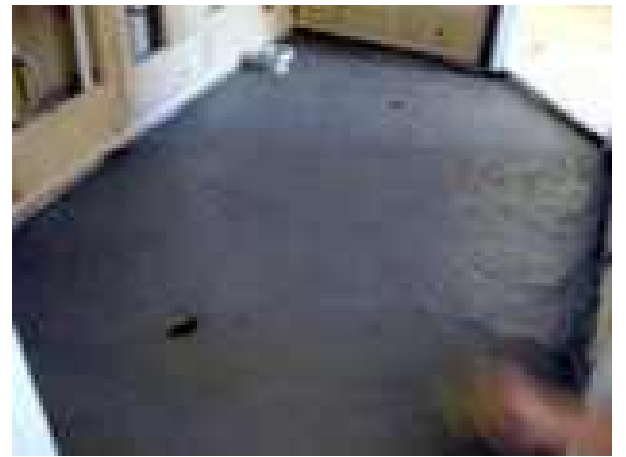
APPLYING A MODIFIED CEMENT SCREED TO SMOOTH OUT THE FLOOR
