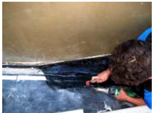
HOT AIR WELDING THE MEMBRANE PARTS TOGETHER
