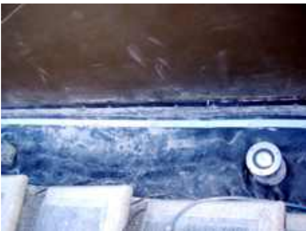
PVC MEMBRANE INSTALLED DETAIL WELDING NEXT
