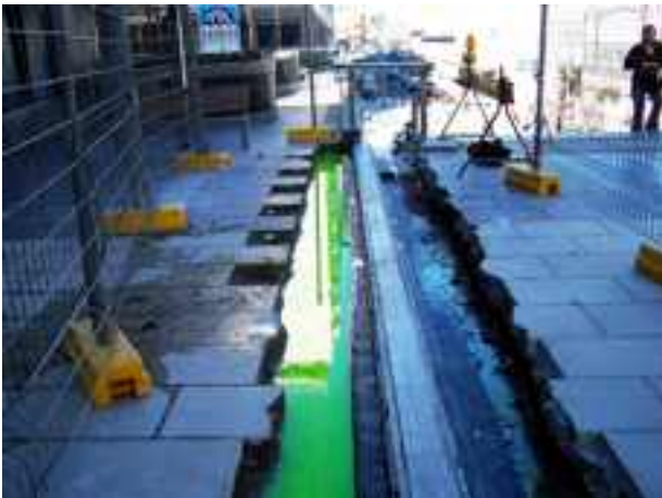
PVC MEMBRANE INSTALLED DETAIL WELDING NEXT
