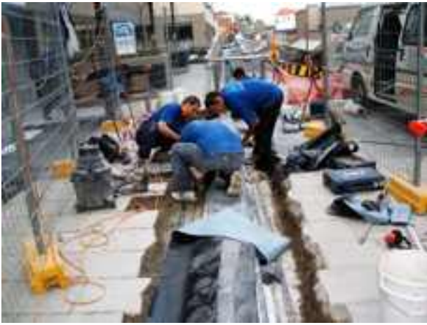
PROPER MEMBRANE TERMINATION REPLACES THE BLOB
