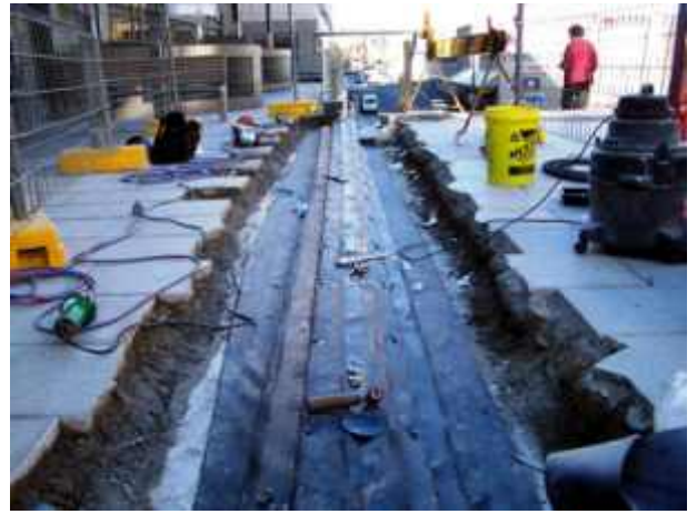
THE EXPANSION JOINT COVER PLATE IS BOLTED BACK IN POSITION
