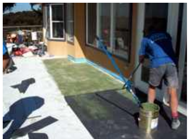
WE DECIDED WE WOULD BOND THE PVC MEMBRANE TO THE SUBSTRATE
