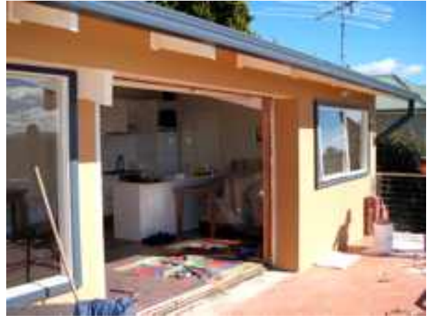
FIRST STEPS REMOVE DOORS AND FRAMES
