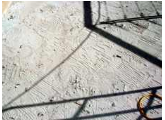
WE DECIDED WE WOULD BOND THE PVC MEMBRANE TO THE SUBSTRATE
