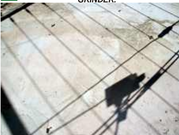
INTO A SMOOTH UNIFORM SURFACE BY GRINDING WITH A DIAMOND FACED GRINDER.
